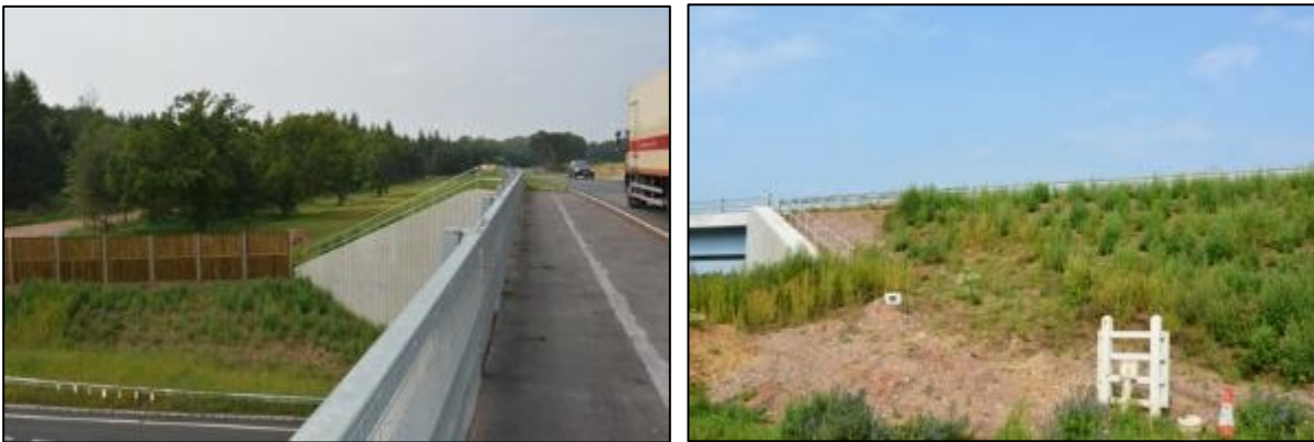
Figure E22. Right: the south east embankment approaching the overbridge, left: treelines/woodland approaching the road and fencing on the north west side of the overbridge.
