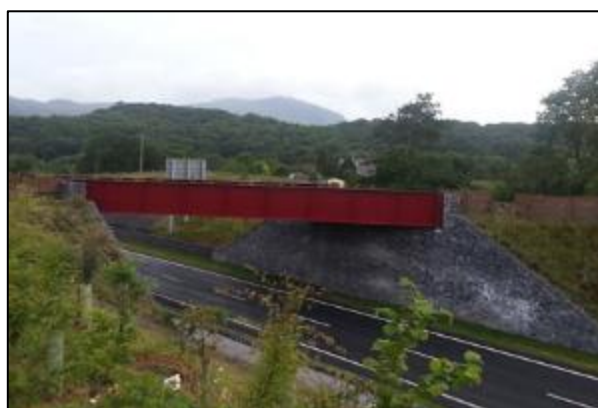
Figure E2. The environmental overbridge on the A487 from the southeast verge.
