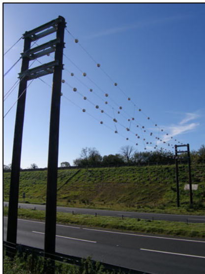
Figure E23. A bat wire bridge on the A590 in Cumbria, England, with the wire and ball design.
